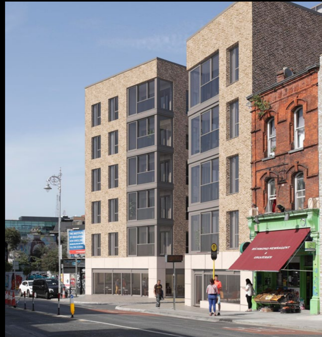
Richmond Street South Entrance Retail Units
