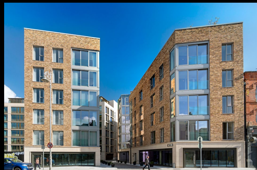
Richmond Street South Entrance Retail Units
